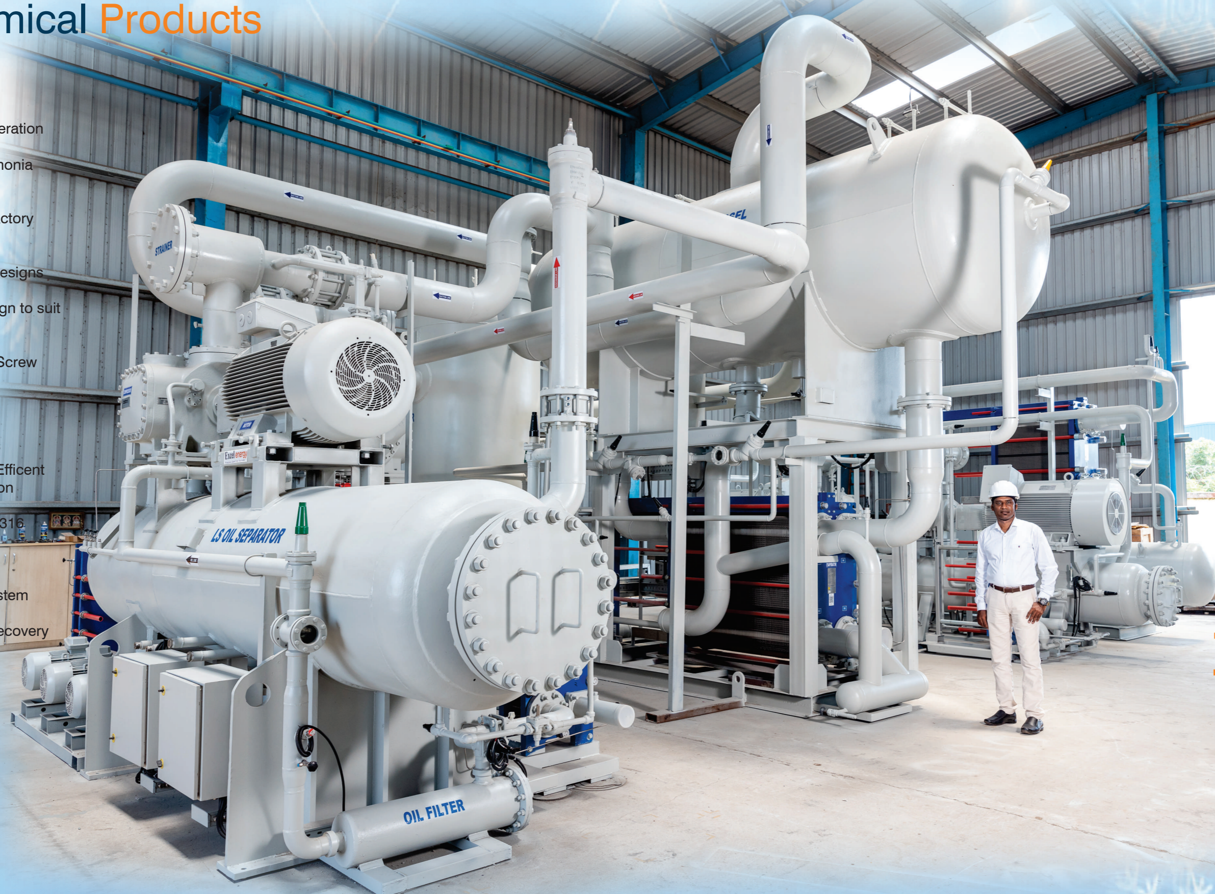
400 TR / Minus 30° C Two Stage Ammonia Refrigeration System for Brine Chilling
